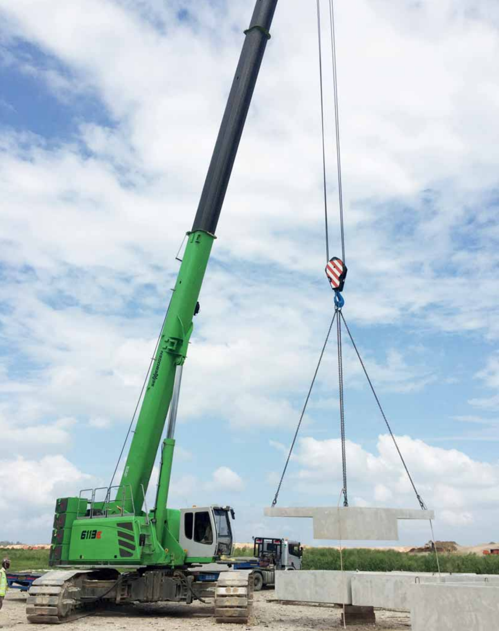
6113 R - Lifting and handling of heavy concrete parts; Singapore
