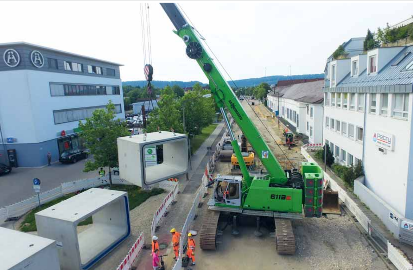
26 6113 R - moving and positioning large and heavy components in civil engineering; Germany
